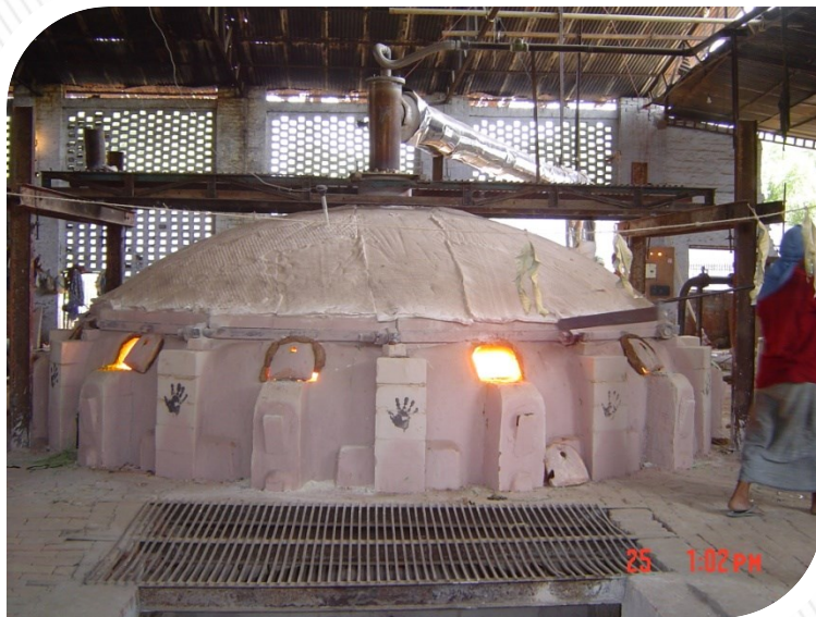
Recuperative natural gas fired pot furnace
