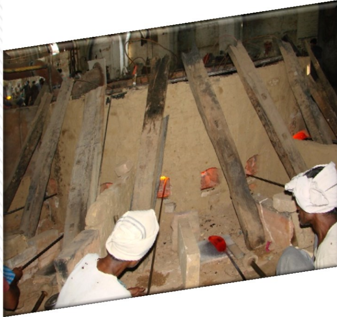
Natural gas fired converter reheating furnace
